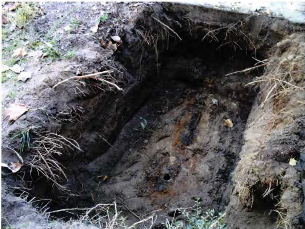
Picture 2: Tank excavation in progress.
